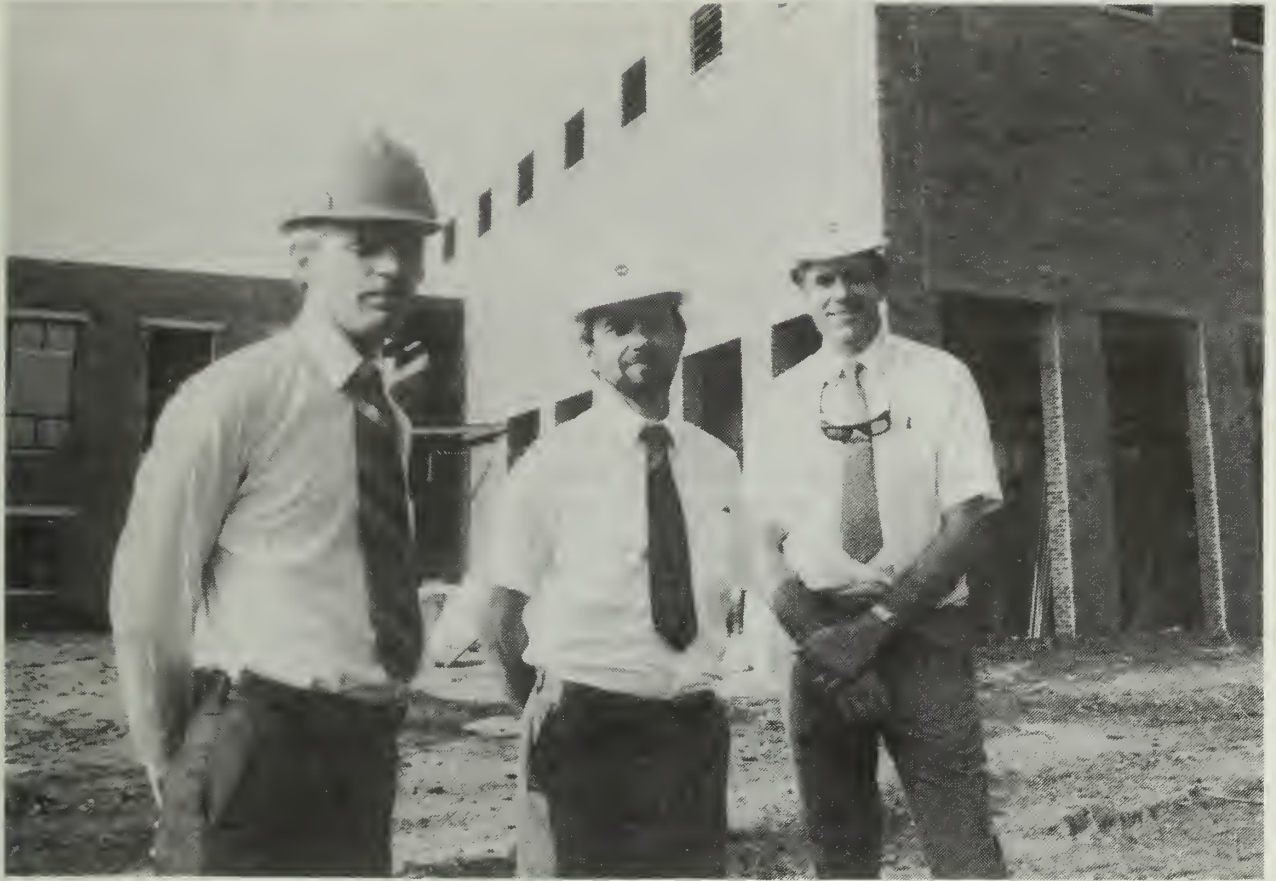
HWRIC Director Dr. David L. Thomas (right), Laboratory Services Program Manager Dr. Marvin D. Piwoni (middle), and Assistant Director Dr. Gary D. Miller inspect construction of the Hazardous Materials Laboratory.
